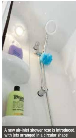
A new air-inlet shower rose is introduced, with jets arranged in a circular shape
