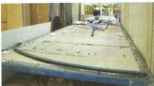
The PU battens are fitted accurately in place using jigsaws
